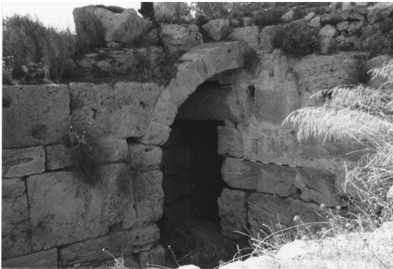
Figure 6.6 View of Entrance to Tower 15 of the Fortress Showing Column Drum Used as Lintel Block
