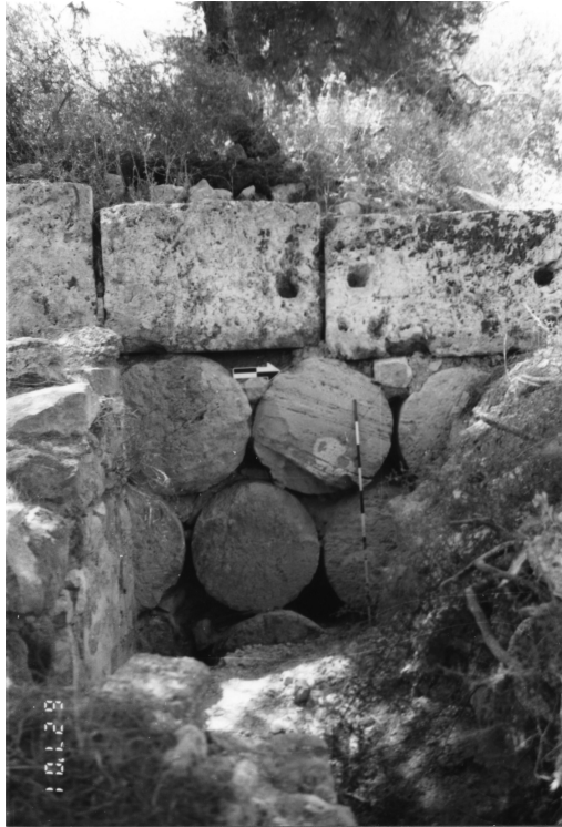
Figure 6.7 Section of Hexamilion Wall ca. 5 Meters North of Roman Bath Showing Use of Spolia
